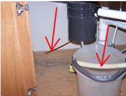
Photo 32 Dishwasher line not attached
